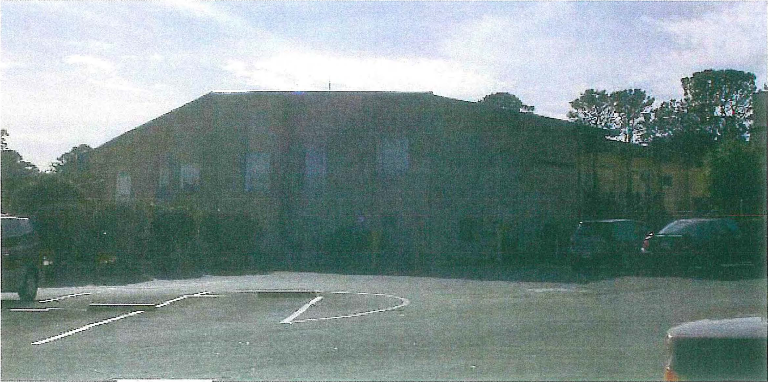
BEFORE: EXISTING ADMINISTRATION BUILDING AND ENTRANCE
